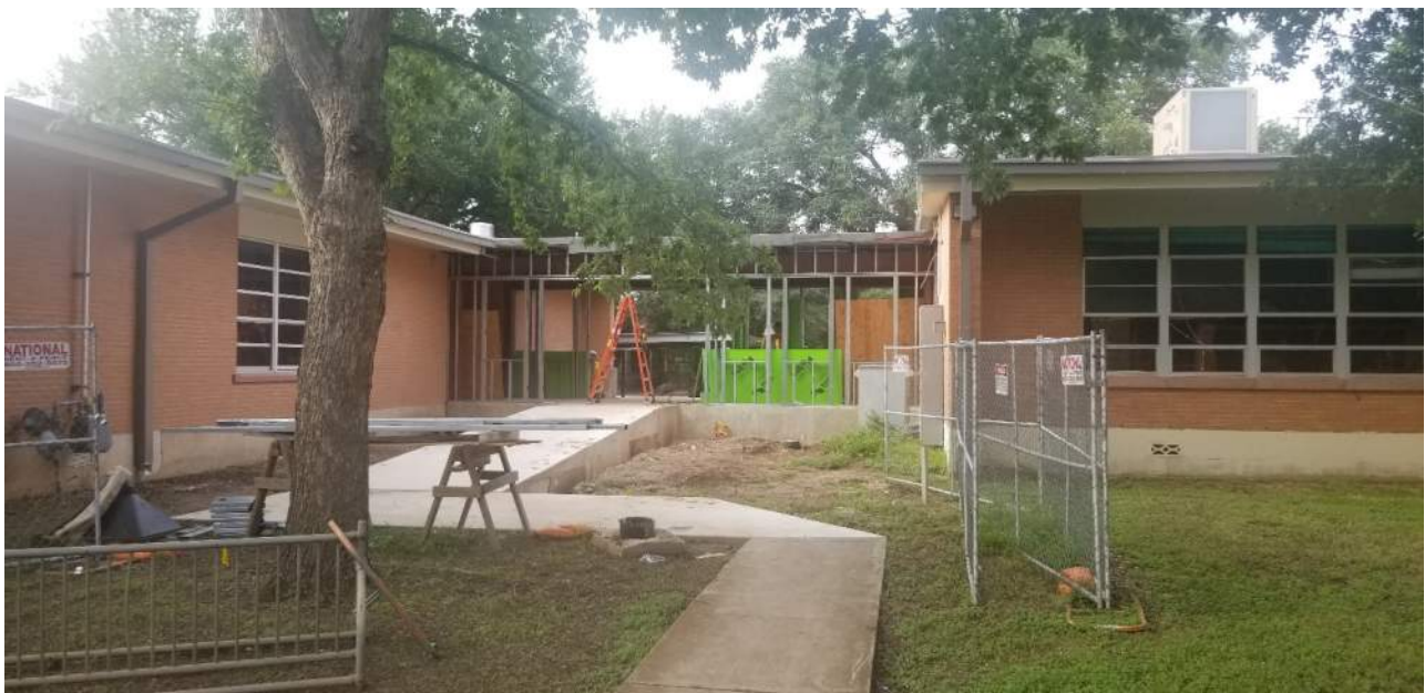
Connector Building and Ramp – view from courtyard
