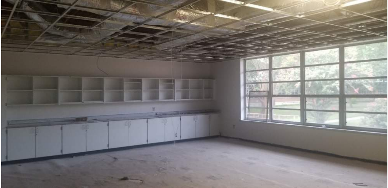
Segment C (Classroom) – Ceiling grid and air registers
