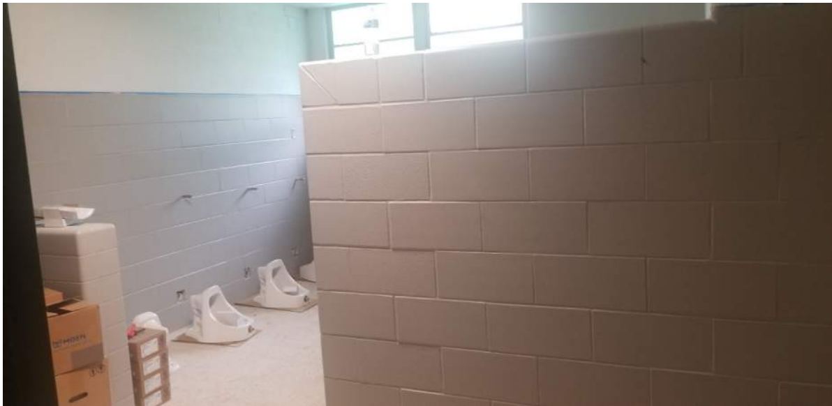
Segment A – Boys Restroom
