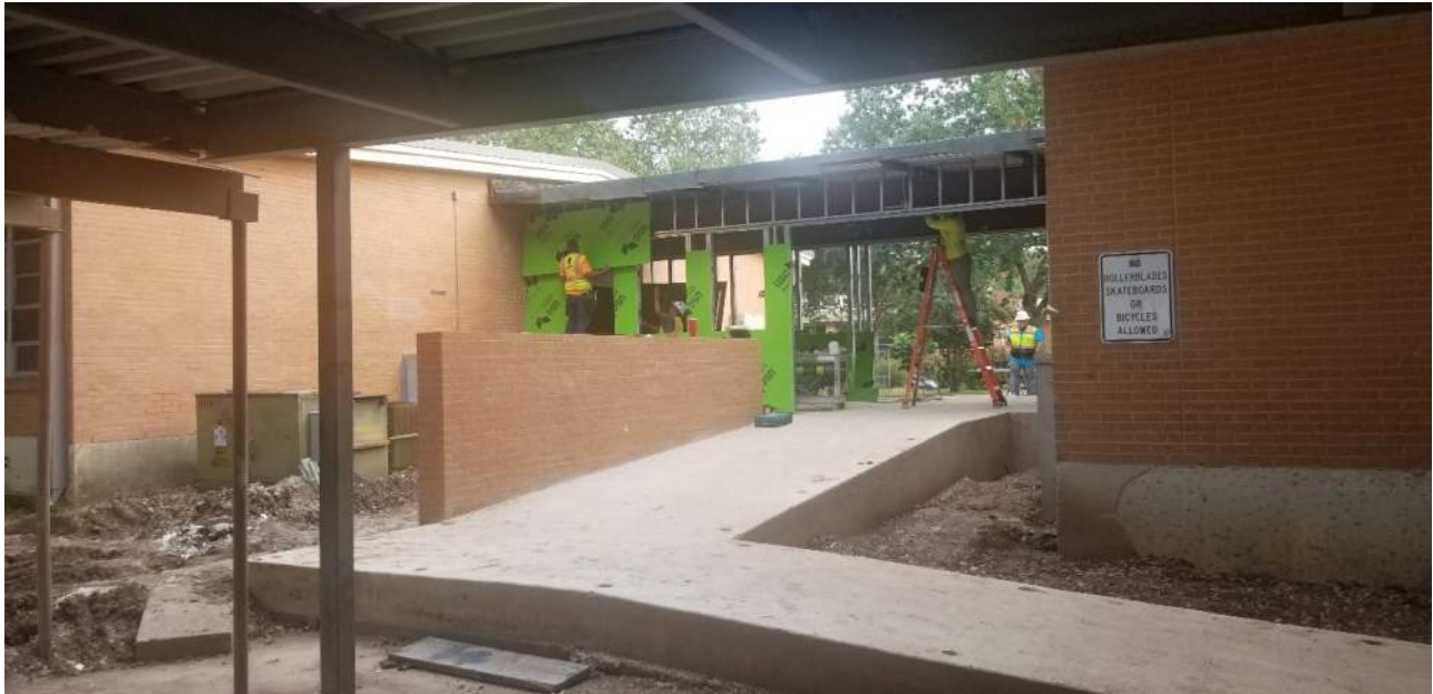
Connector Building and Ramp – working on exterior wall framing
