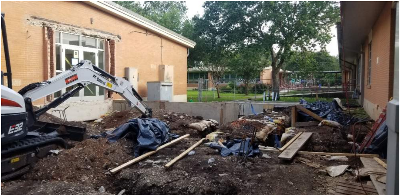
Conneting Structure – Foundation work on hold due to rain
