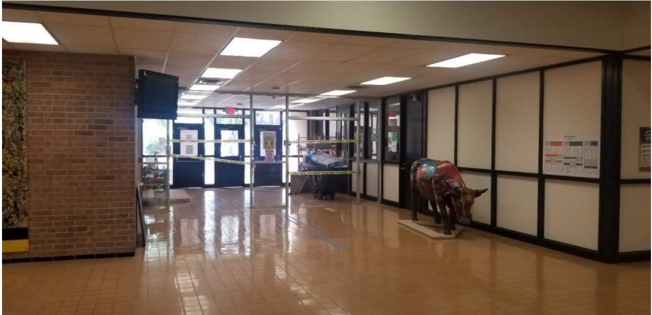
Demolition at existing secured vestibule
