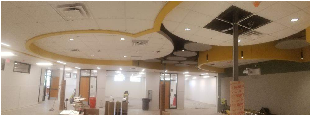
Segment D (7 th Grade Wing) – Collaborative Area Ceiling
