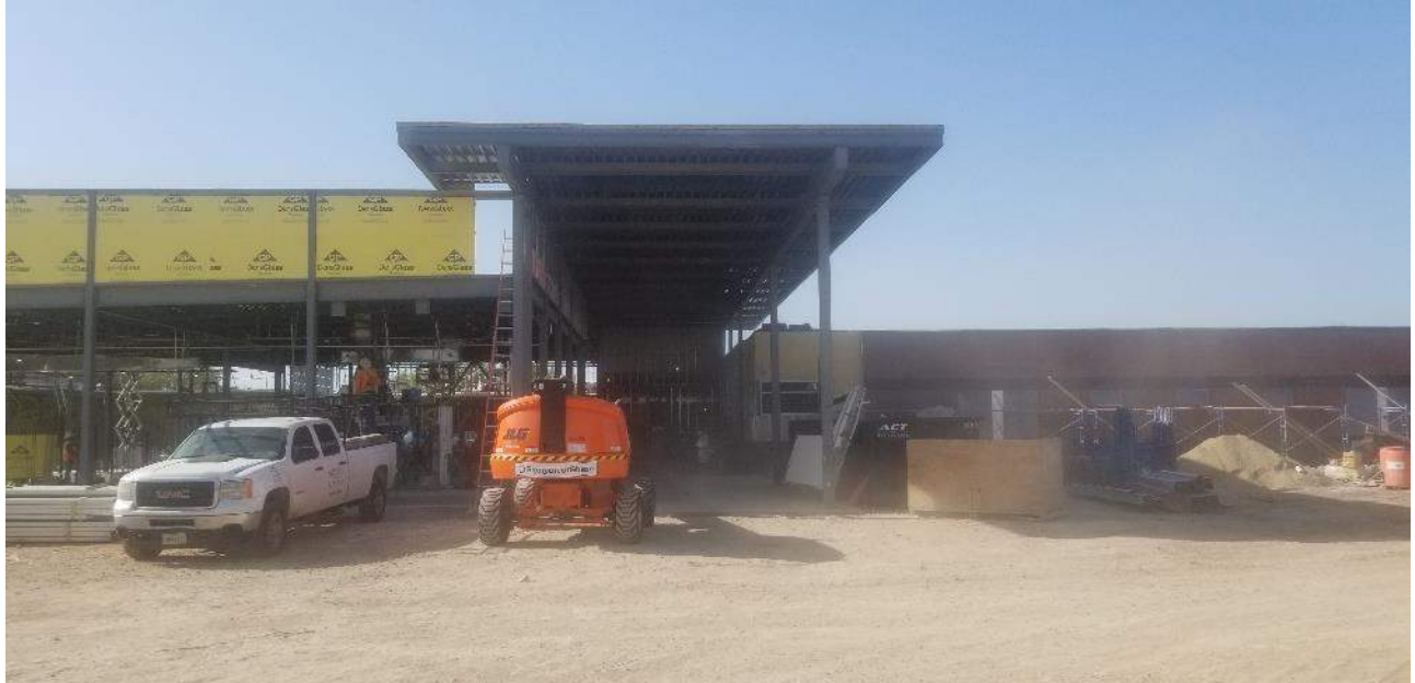
Segments F & H (8 th Grade Wing & Kitchen) – Structural framing at main entrance to cafeteria from Bus Loop
