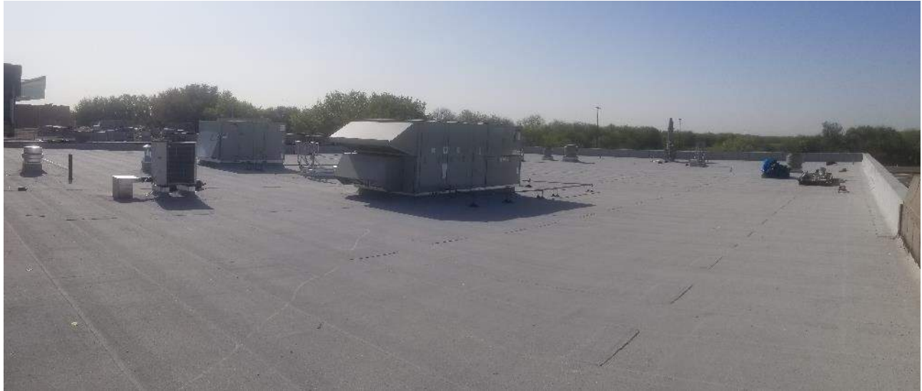
Segment F (8 th Grade Wing) – Material and debris left on new roof
