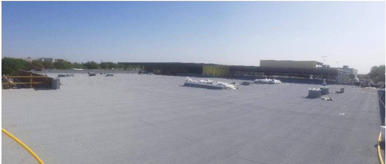
Segment F (8 th Grade Wing) – Material and debris left on new roof
