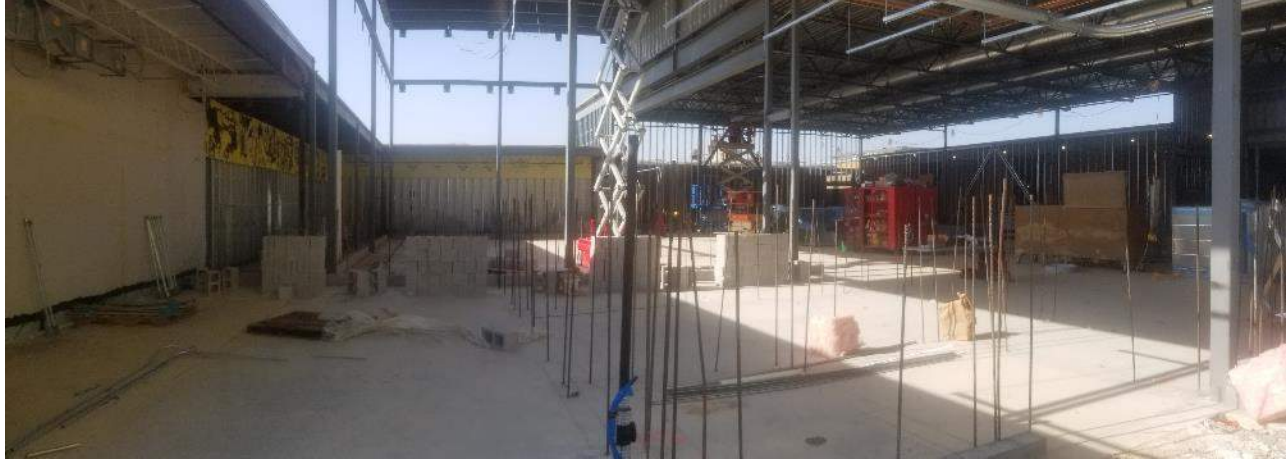
Segment G (Cafetorium) – CMU work at platform area
