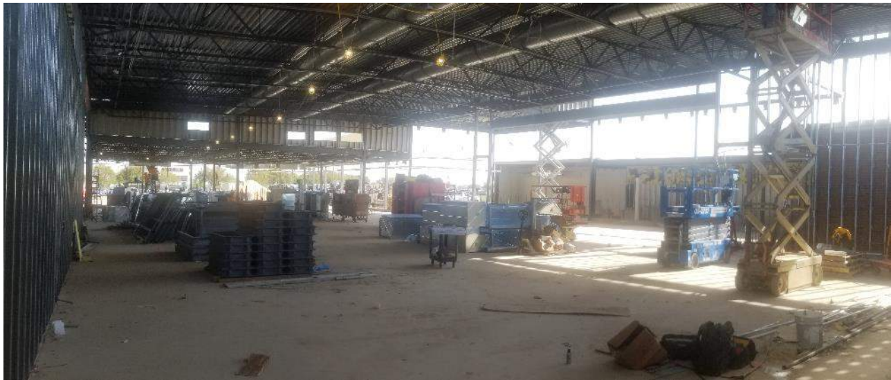
Segment G (Cafetorium) – Exterior wall framing and overhead MEP
