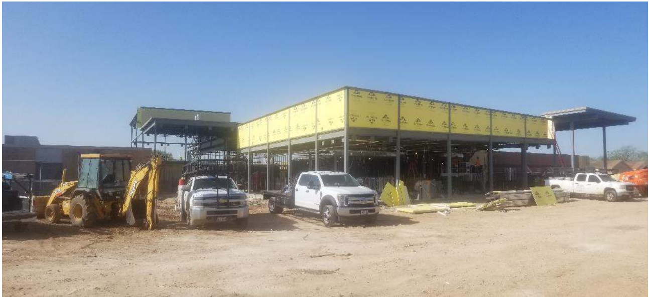
Segments G & H (Kitchen & Cafetorium) – Structural framing, exterior framing and sheathing
