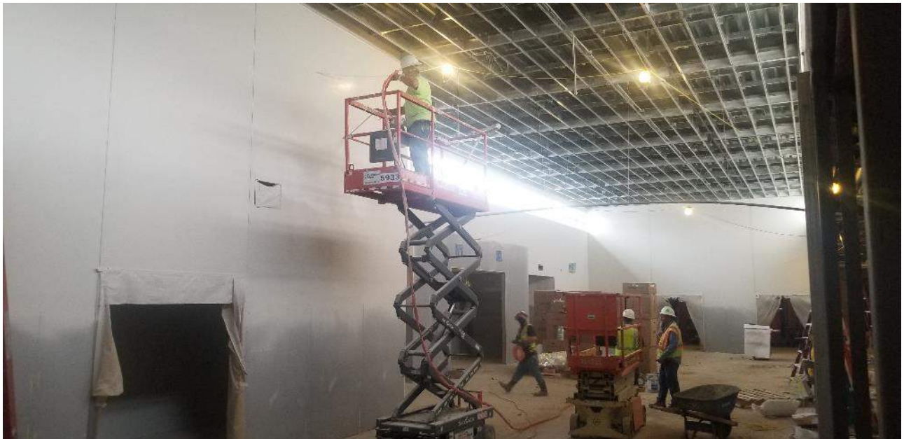
Segment D (7 th Grade Wing) – Central Corridor
