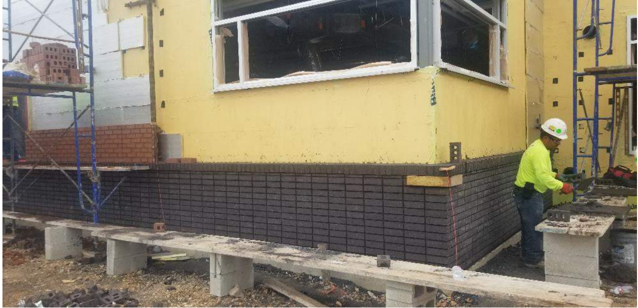
Segment D (7 th Grade Wing) – Brick veneer
