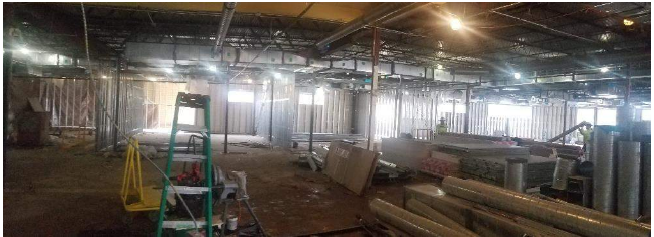
Segment F (8 th Grade Wing) – Interior framing
