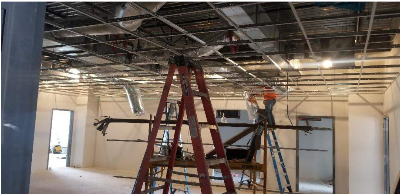
Segment D (7 th Grade Wing) – Science Classroom ceiling grid installation
