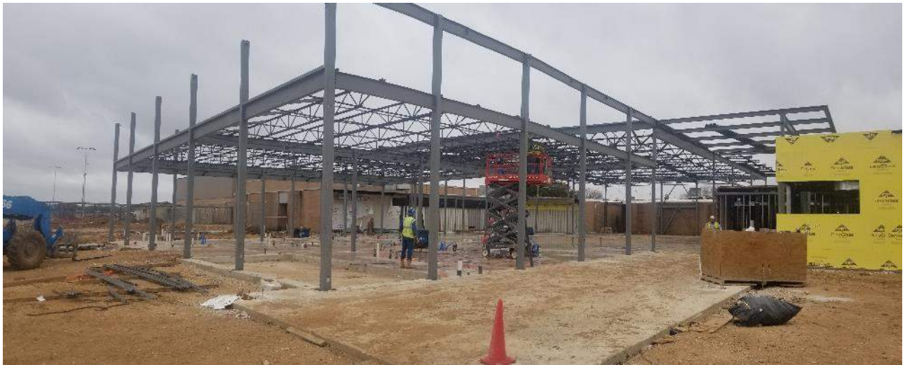
Segments F & G (8 th Grade Wing & Cafetorium) – Structural framing
