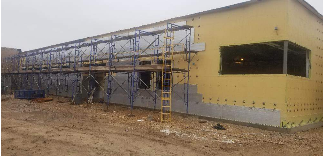
Segment D (7 th Grade Wing) – Exterior waterproofing and rigid insulation board
