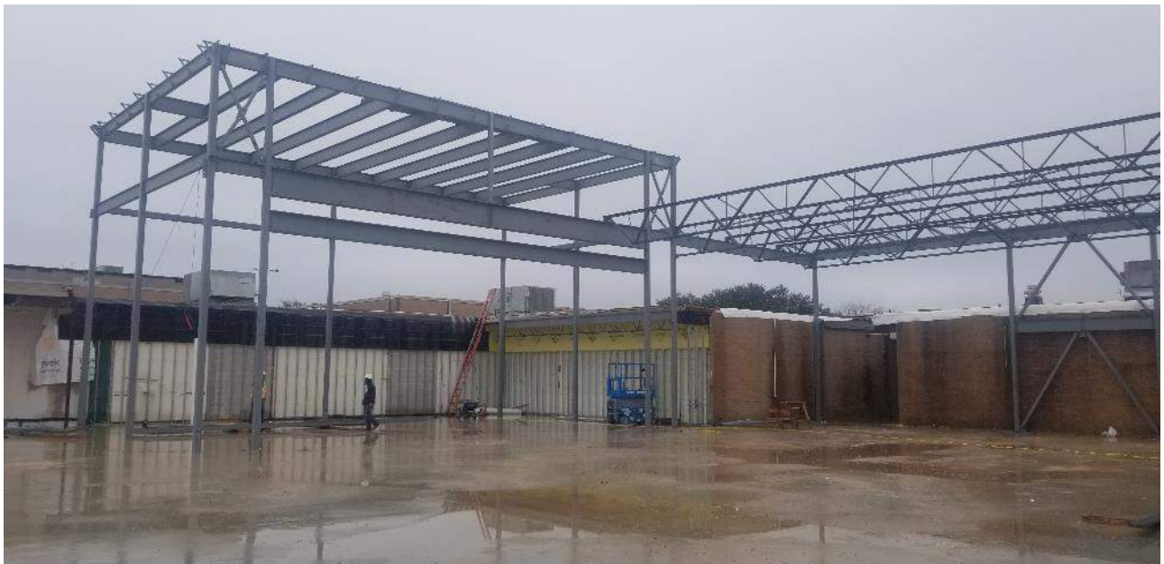
Segment G (Cafetorium) – Structural framing of Stage
