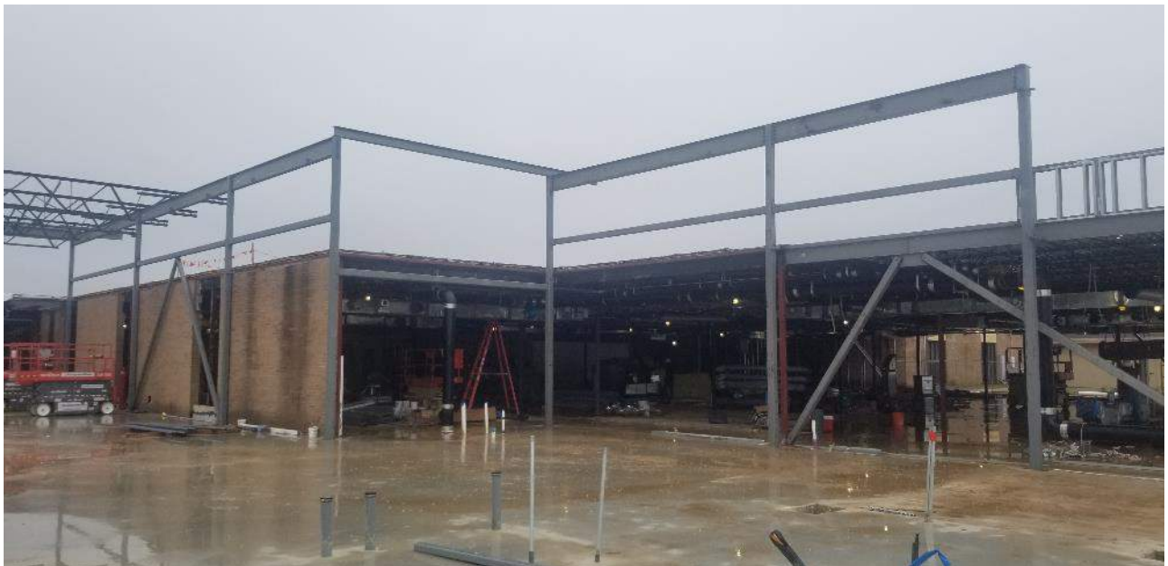
Segments F & G (8 th Grade Wing & Cafetorium) – Structural framing
