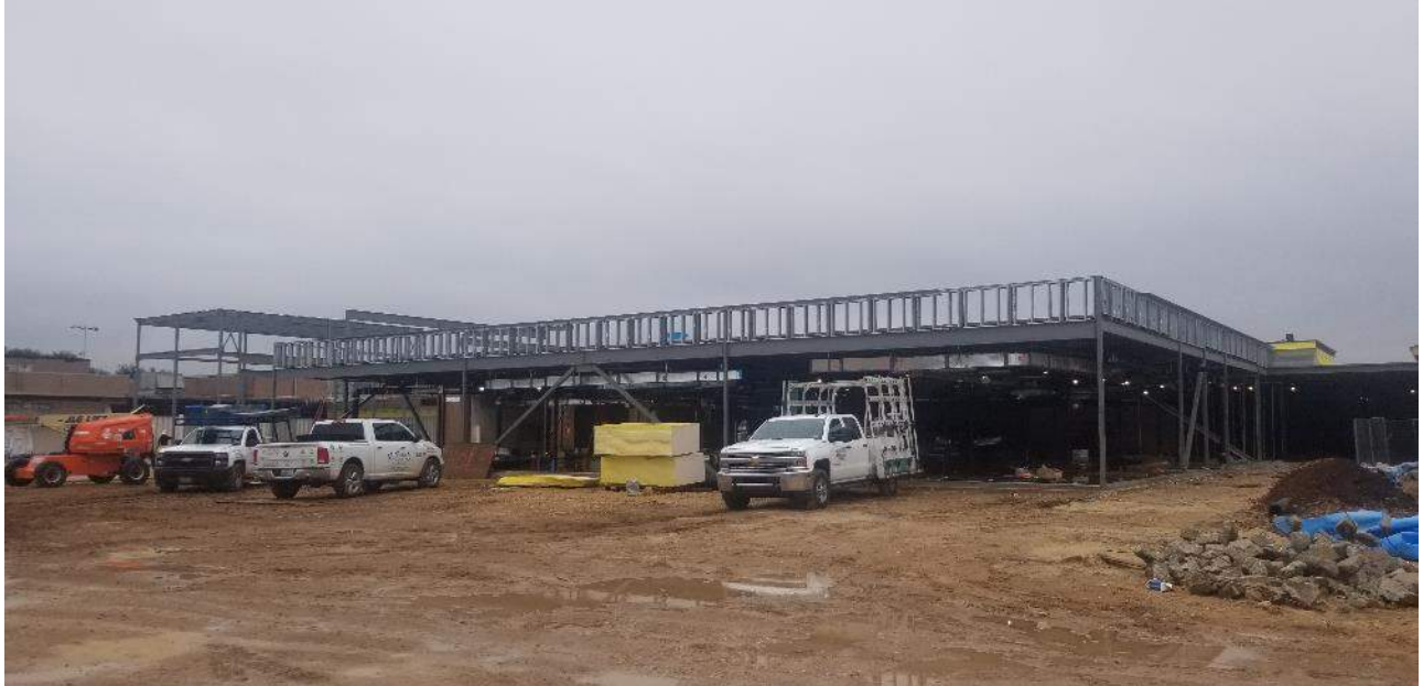
Segment F (8 th Grade Wing) – Exterior parapet framing
