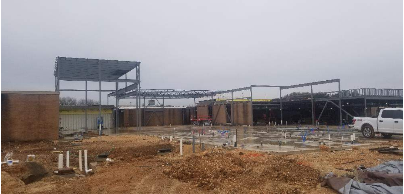
Segments G & H (Kitchen & Cafetorium) – Structural framing
