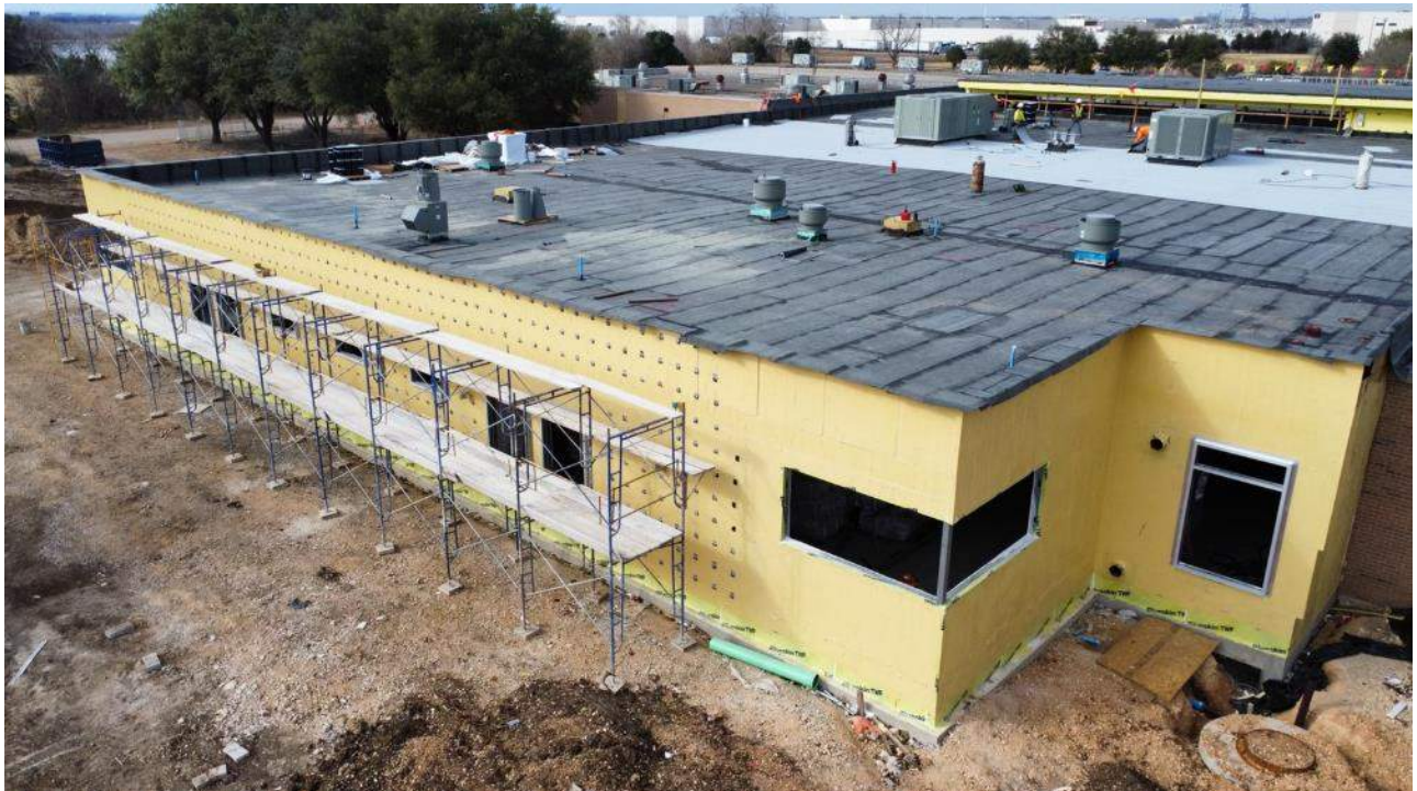
Segment D (7 th Grade Wing) – Roofing and RTU's (roof top units)
