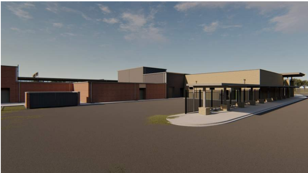
View of Service Drive and Bus Canopy
