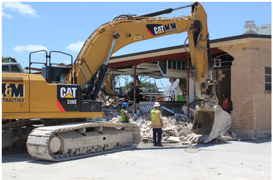
Major demolition work began during summer 2015 on the new Seguin High School construction project.
