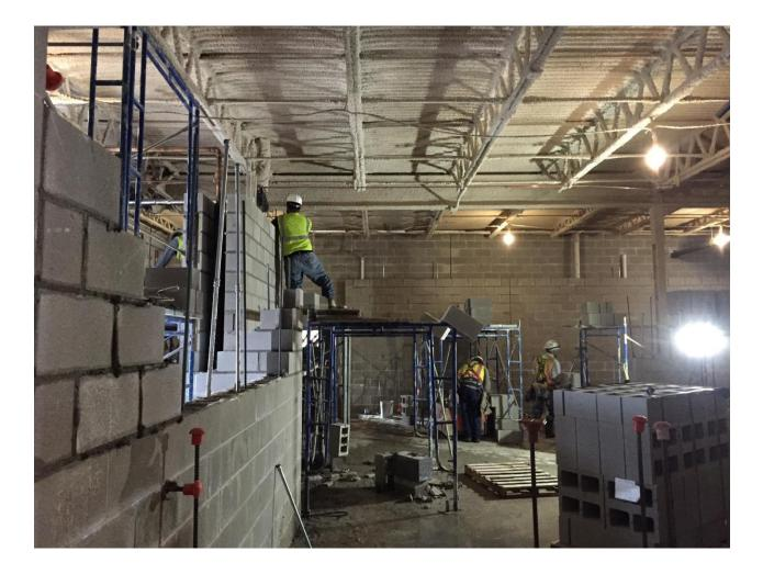
**ATHLETICS** – Sprayed on fireproofing of the steel structure has been completed. Interior block work installation continues.
