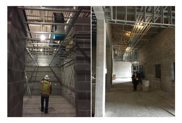
**GYMNASIUM AND ATHLETICS DEPARTMENT** – Metal stud framing for ceiling furr outs is being installed. Ductwork and above ceiling MEP work are in progress.
