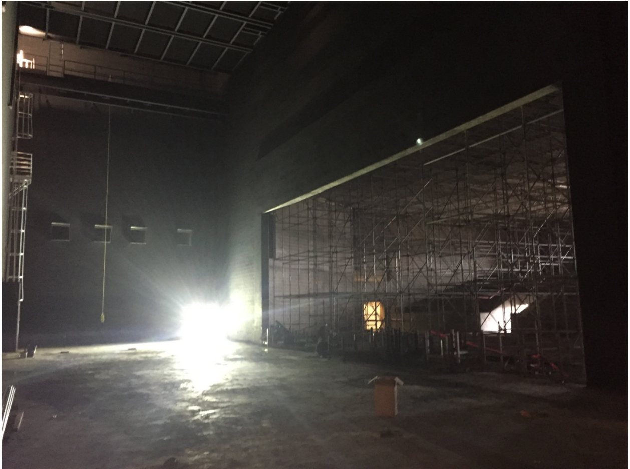
PERFORMING ARTS CENTER – Final coat of paint at Fly-loft, in area A.
