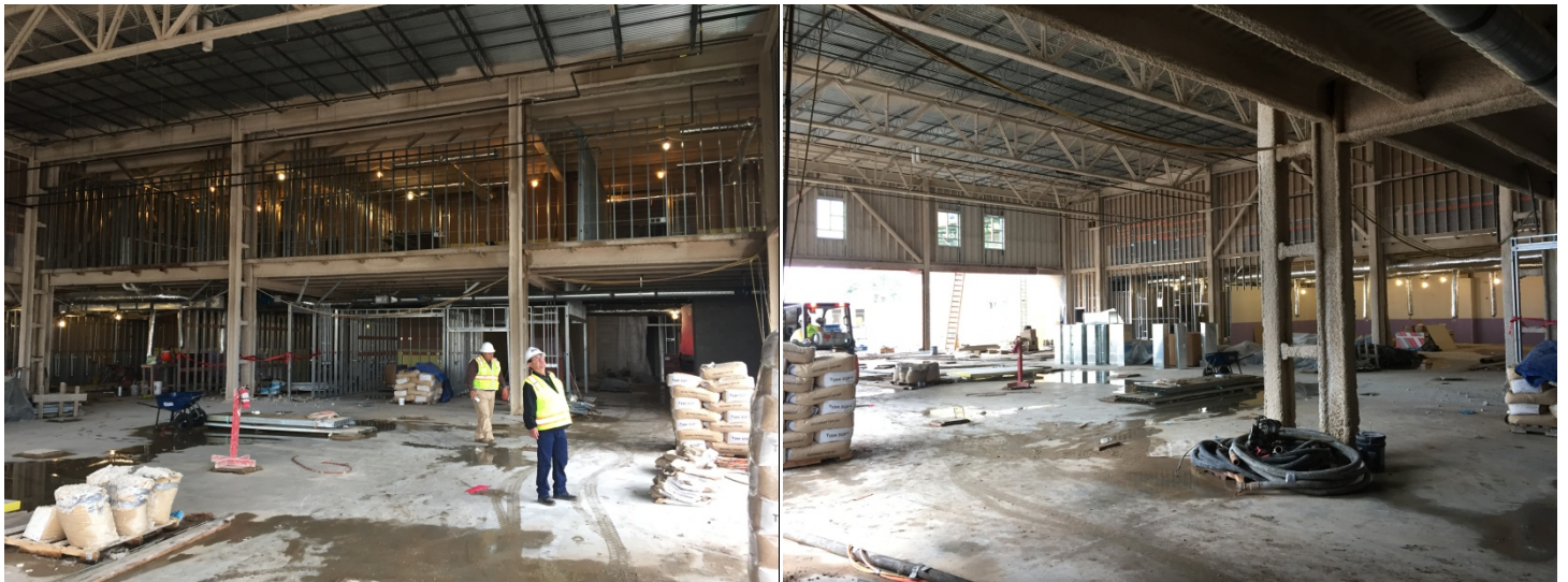
LIBRARY – On-going interior drywall framing (left photo). On-going exterior drywall framing and sheathing work (right photo).
