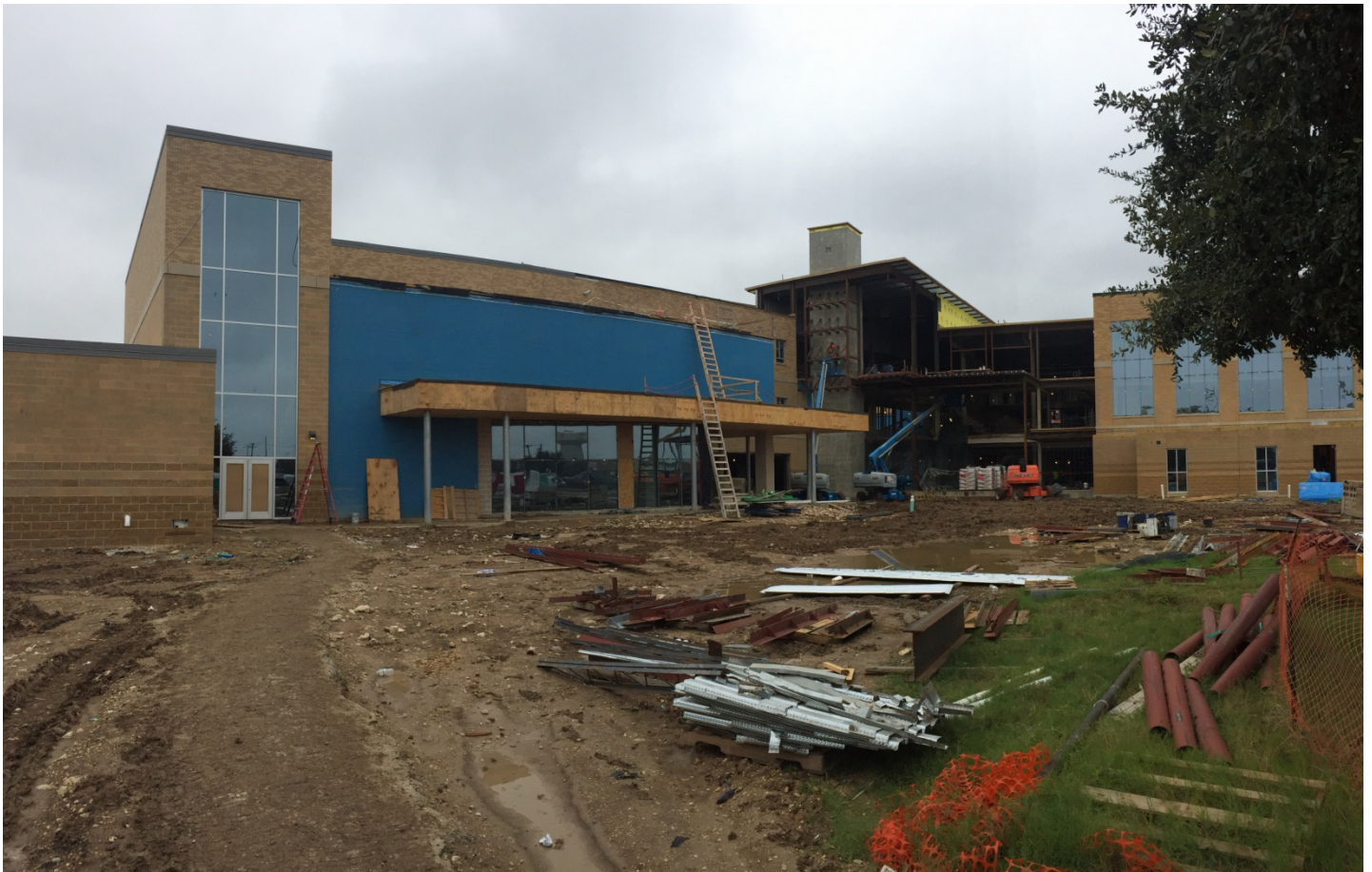
NORTH VIEW OF MAIN ENTRANCE TO SCHOOL On-going miscellaneous work throughout.
