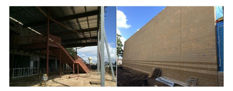
PERFORMING ARTS CENTER - Structural steel erection, and roof decking at lobby of PAC (left photo). Block veneer going up, around the north and west facades of the PAC. (Right photo).
