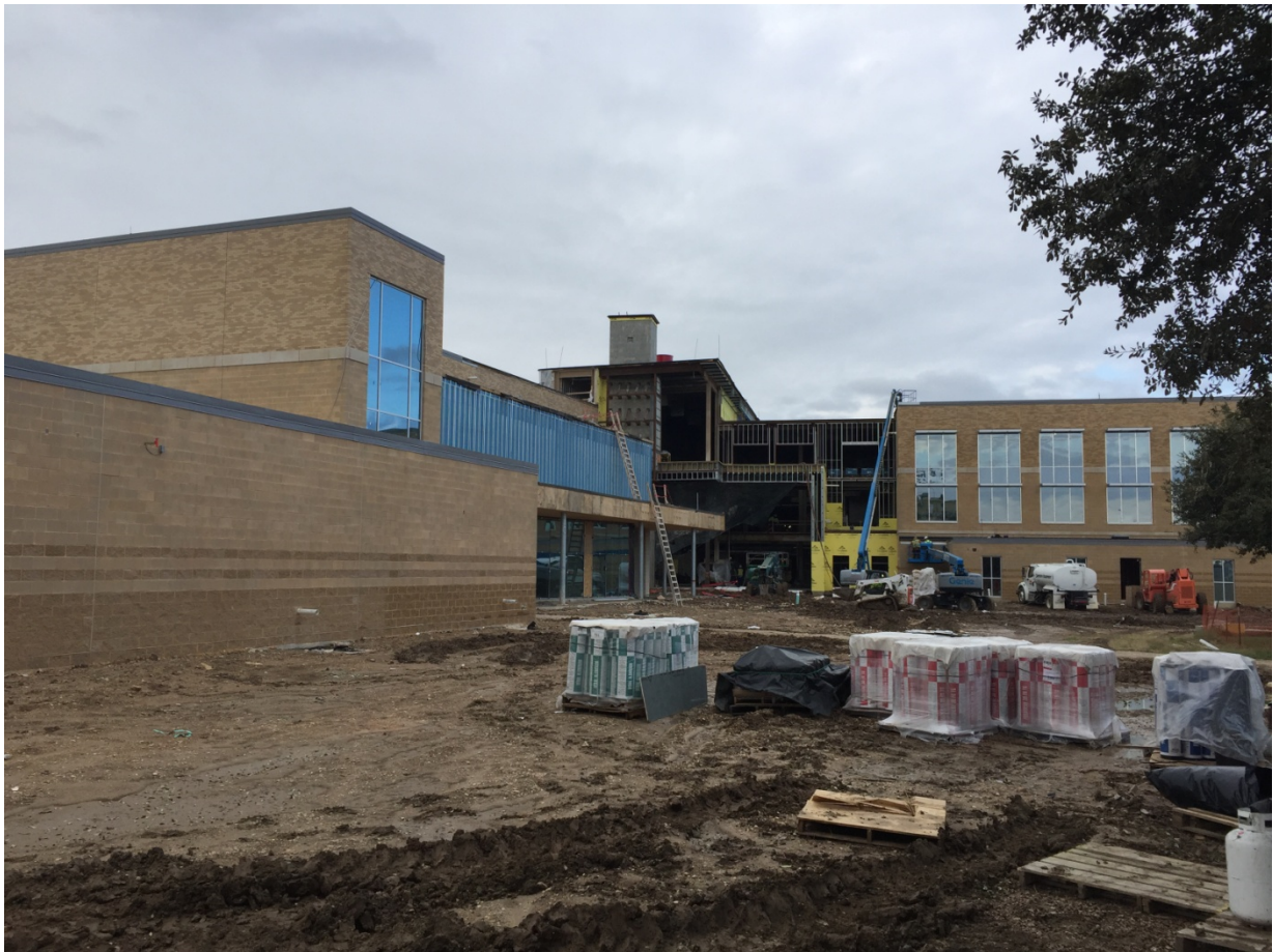
NORTHEAST VIEW OF MAIN ENTRANCE TO SCHOOL On-going miscellaneous work throughout.
