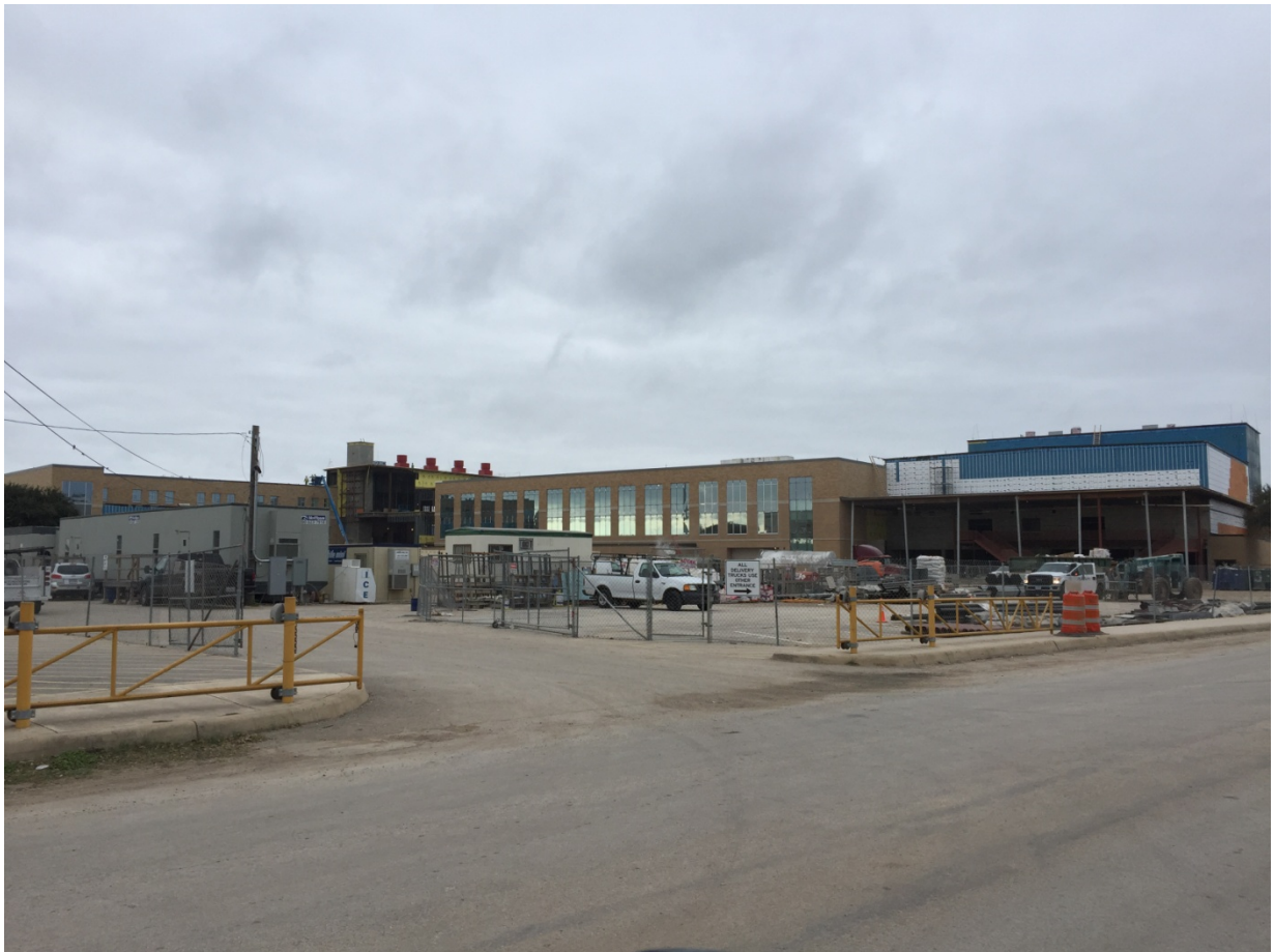
NORTH EAST VIEW OF SCHOOL On-going miscellaneous work throughout.
