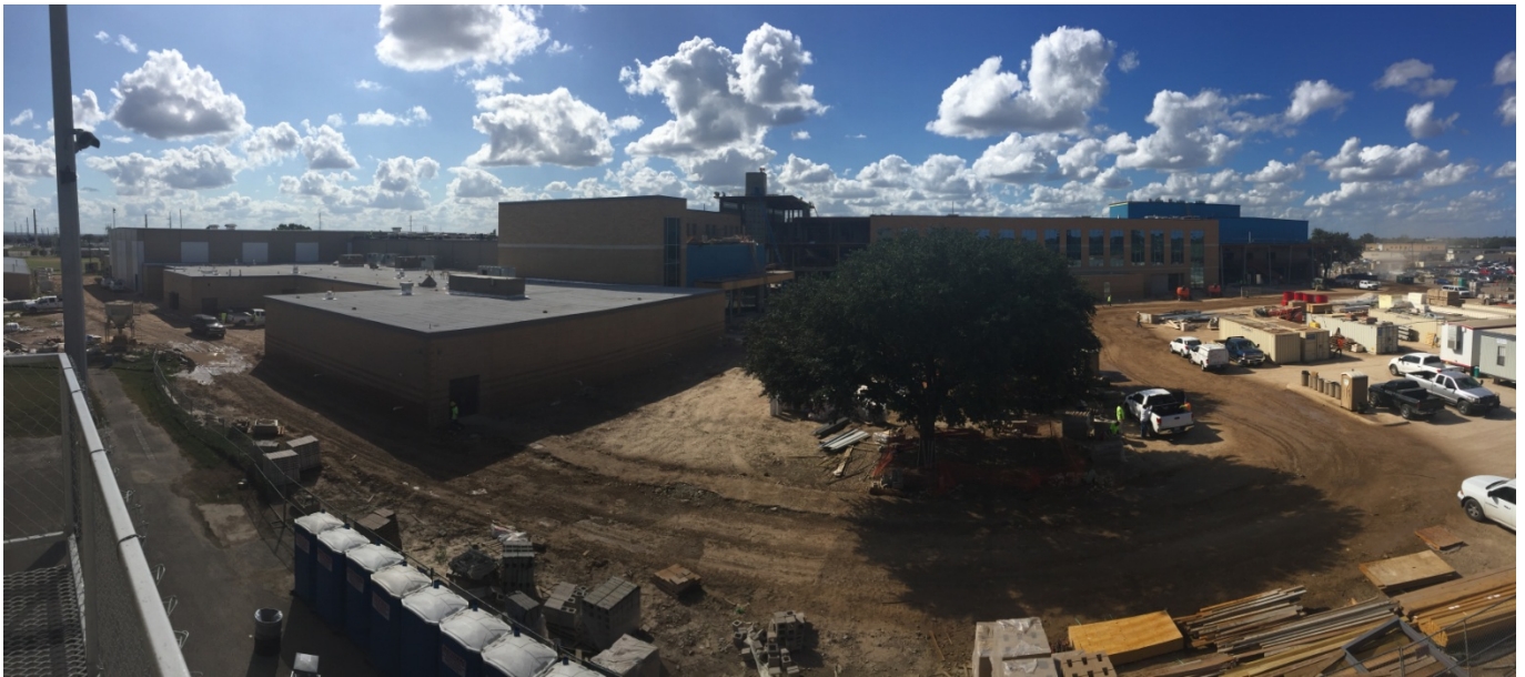
BIRDSEYE VIEW OF PROJECT SITE FROM PRESS BOX On-going miscellaneous work throughout.
