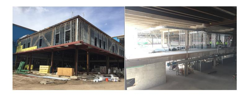
**LIBRARY** – Light gauge metal studs framing of exterior walls in progress (left photo). Drywall framing of support spaces, adjacent to main atrium. (Right photo).
