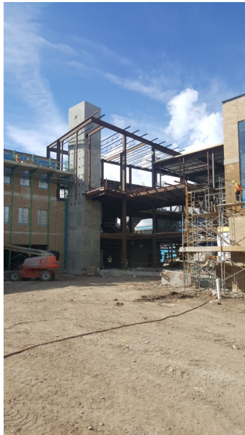
VIEW OF MAIN ENTRANCE TO THE SCHOOL (ELEVATOR/CLOCK TOWER) On-going steel detailing and MEP work.
