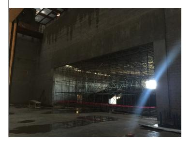
**PERFORMING ARTS CENTER** – On-going MEP work in all corridors. Block filler application in progress (left photo). Scaffolding in place, for work performed above auditorium seating area. (Right photo).
