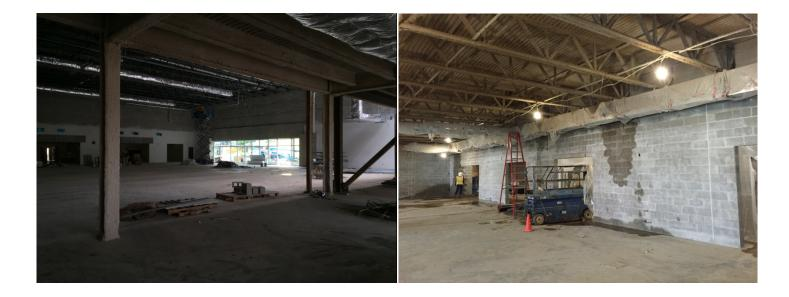
**CAFETERIA** – On-going MEP work, and curtain wall installation in dining area (left photo). Sprayed-on fireproofing application, in kitchen area. (Right photo).
