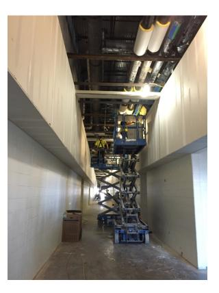
**INTERIOR** – Ceramic wall and floor tile installation, and shower units at wet walls in Athletic areas (left photo). Drywall and mechanical work at hard ceilings in Athletic corridor, between gymnasiums. (Right photo).
