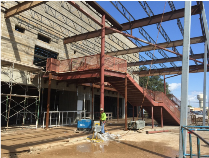
PERFORMING ARTS CENTER – Structural steel erection at lobby of PAC (left photo). On-going erection of scaffolding above the seating area, in the Auditorium (right photo).
