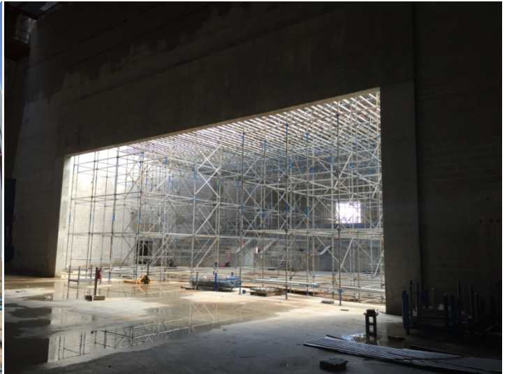
PERFORMING ARTS CENTER – Structural steel erection at lobby of PAC (left photo). On-going erection of scaffolding above the seating area, in the Auditorium (right photo).
