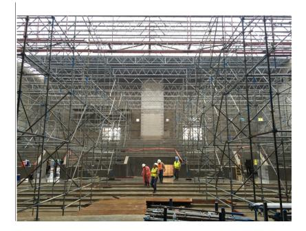
**PERFORMING ARTS CENTER** – On-going work at the roof level, above back of house corridor (left photo). On-going steel detail work above the seating area, in the Auditorium (right photo).
