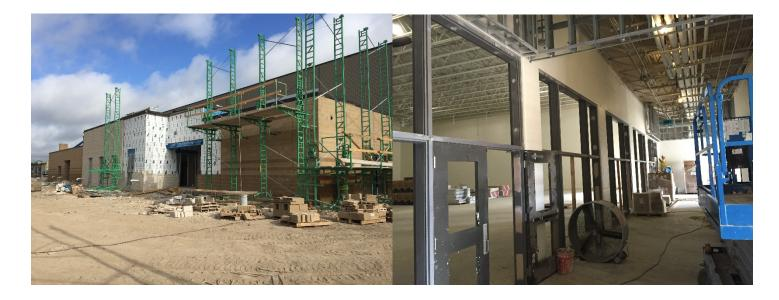
**INTERIOR** – The photograph on the left shows the installation of the block veneer at the south end of the gymnasiums (Lobby, Restrooms, and support spaces). The photograph on the right shows continuing work on hollow metal frames/doors installation at the Athletic Lobby (south of the gymnasiums).
