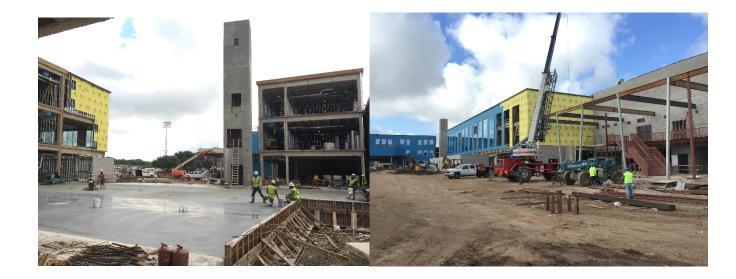
**ELEVATOR / CLOCK TOWER and PERFORMING ART CENTER** – Poured last portion of foundation at area F, adjacent to Clock Tower (left photo). Structural steel erection of Performing Art Center lobby area (right photo).
