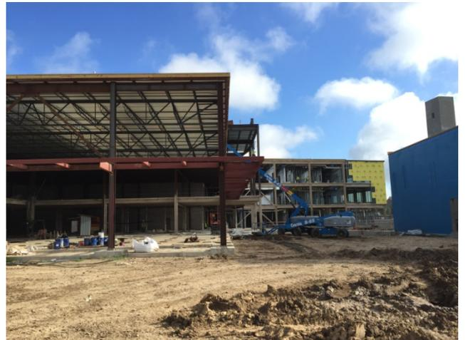
**ELEVATOR / CLOCK TOWER and FUTURE COURTYARD** – Working on foundation forms at/around tower and courtyard (along Area F). The elevator/clock tower construction continues this week.
