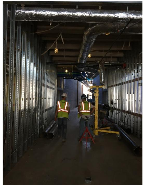
**INTERIOR** – The photograph on the left shows the 3 story connection to the existing Freshman Center. The photograph on the right shows continuing work on metal stud interior walls, ductwork and electrical, at Area B corridor, adjacent to the north of the existing Band Hall.
