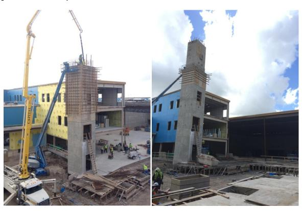
**ELEVATOR AND CLOCK TOWER** – Concrete is being poured on the walls of the new elevator shaft last week. The elevator/clock tower construction continues this week.
