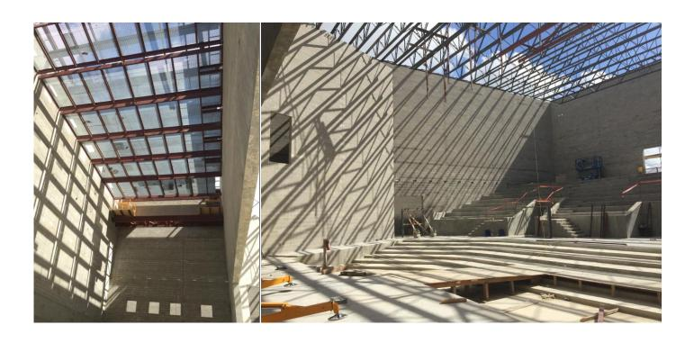
PERFORMING ARTS CENTER – The photograph on the left shows the gridiron platform above the stage. The photograph on the right shows on-going block installation at the interior side wall of the seating area.
