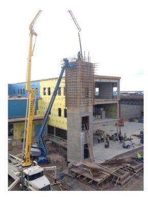
**ELEVATOR AND CLOCK TOWER** – Concrete is being poured on the walls of the new elevator shaft. A new exterior wall clock will be installed at the top of the tower and it will be facing the stadium and Hwy 123.
