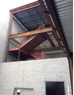
STEEL STRUCTURE - The photographs show the installation of the steel structure above the main corridors and the Library.
