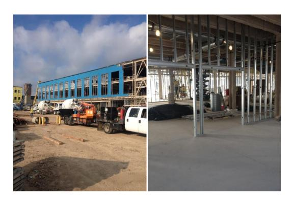
**ADMINISTRATION AND CLASSROOMS** – The photograph on the left shows the site conditions on Tuesday July 7, 2016. Window framing and glass installation is in progress. The photograph on the right shows the interior of the administration area. Ductwork installation is in progress. Some interior metal stud walls have been erected.
