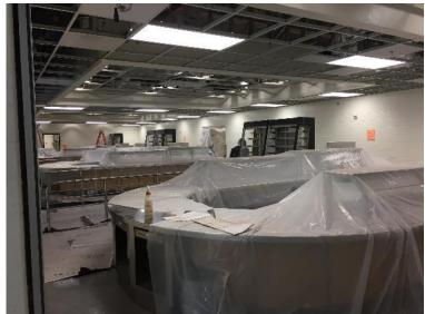
**CAFETERIA/KITCHEN** – Working on above ceiling punch in Kitchen/Serving Lines. (top left photo). Installing ceiling tiles, and prepping surfaces for finishes in Cafeteria. (bottom photo).
