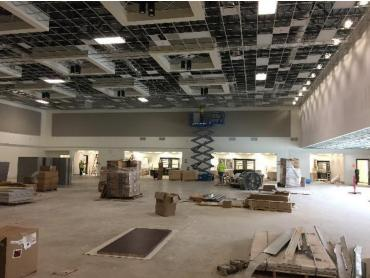
**CAFETERIA/KITCHEN** – Working on above ceiling punch in Kitchen/Serving Lines. (top left photo). Working on above ceiling punch, and prepping surfaces for finishes in Cafeteria. (bottom left photo).
