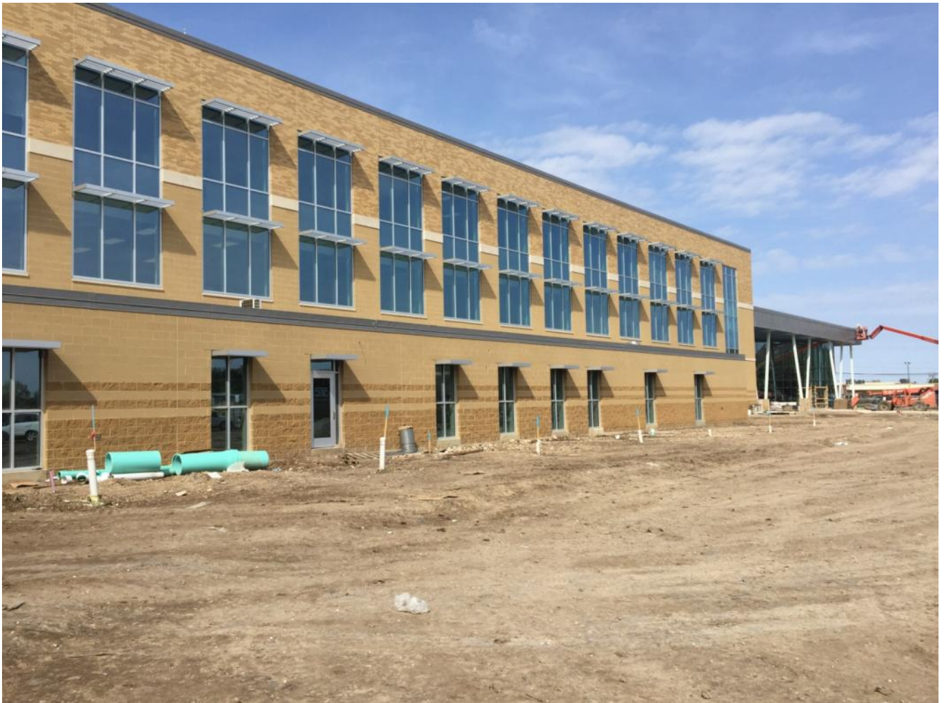
EAST VIEW OF ADMINISTRATION/CLASSROOMS & PAC Site work at main drive / drop-off loop
