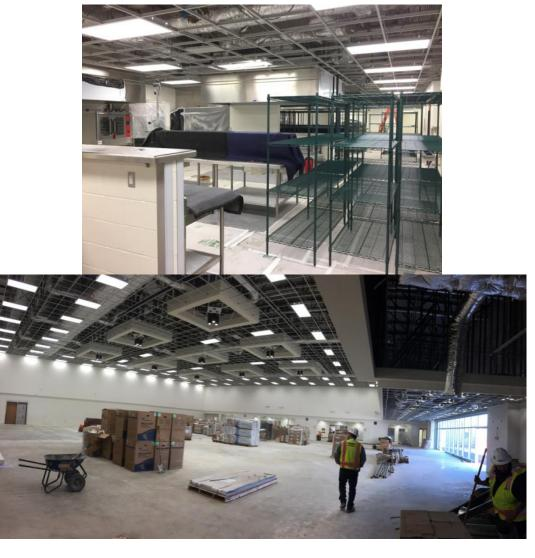
**CAFETERIA/KITCHEN** – Installing food service equipment in kitchen (top photo). Taping and floating drywall, and ceiling grid work in Cafeteria. (Bottom photo).
