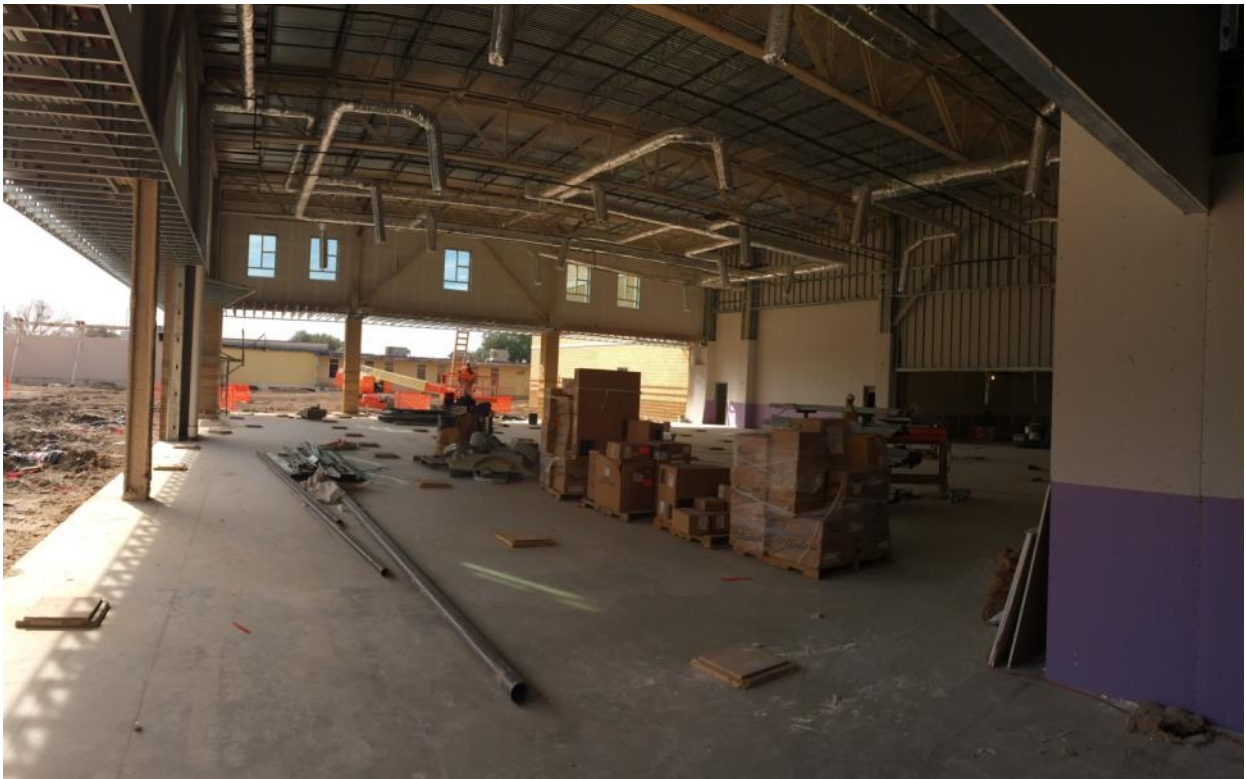
LIBRARY – On-going interior sheetrock work.
