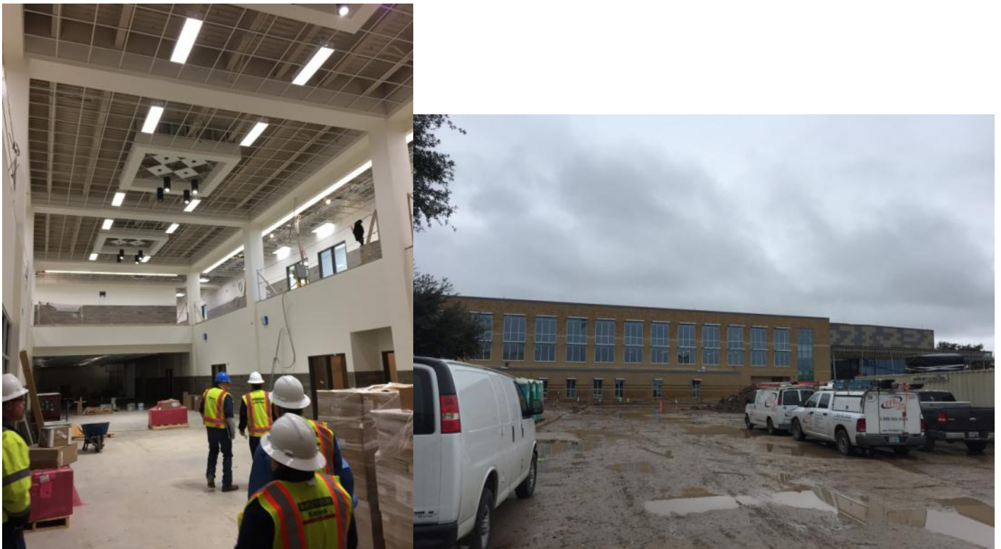
ADMINISTRATION AND CLASSROOMS – Painting of walls, installing speakers, and light fixtures in atrium at the administration and classroom area (left photo). Exterior view of area C. (right photo).
