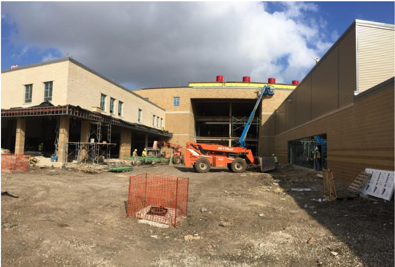
COURTYARD (SOUTH) - located between Library (on left) and Cafeteria (on right) On-going masonry work
