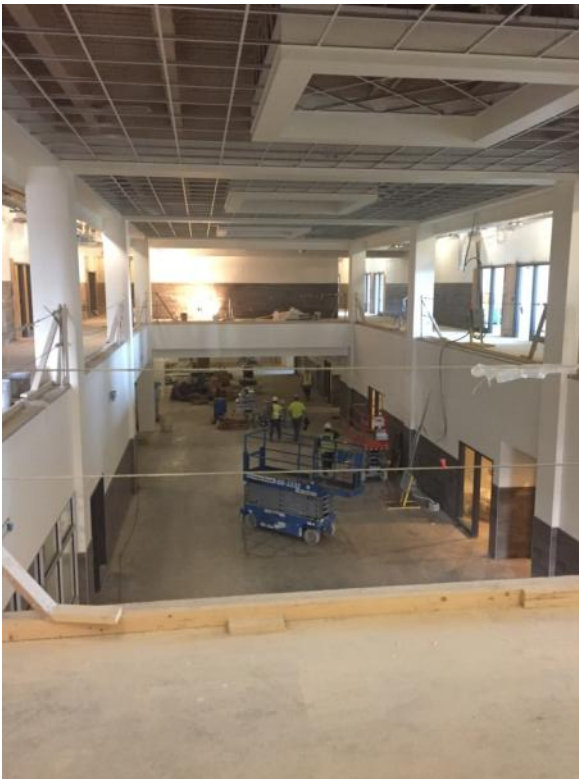
ADMINISTRATION AND CLASSROOMS – Painting of walls in atrium at the administration and classroom area (left photo). Painting of walls and installation of lay-in ceiling grid and light fixtures in a typical classroom (located along the east side of area C). (Left photo).
