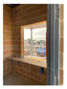
Press Box – Installing metal furring to receive metal panels.
