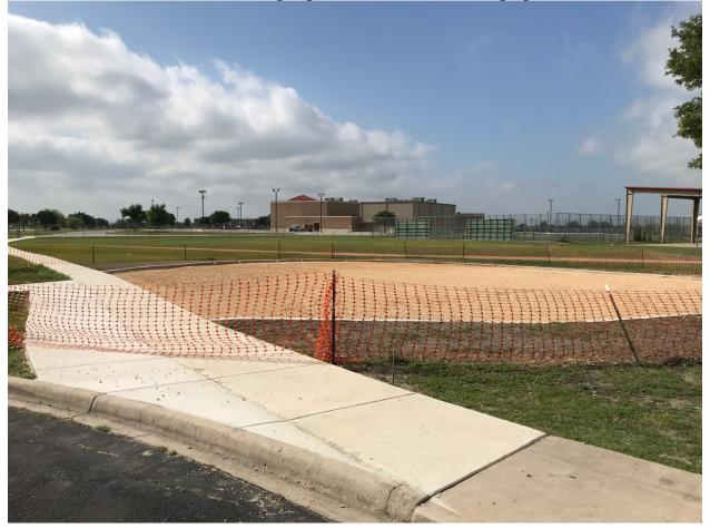
Vogel concrete curbing and sidewalk work is complete. Base material has been added and leveled to prepare the site for the equipment installation.
