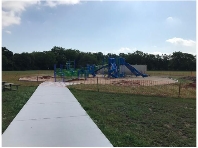
Koennecke concrete curbing and sidewalk work is complete. Base material has been added and leveled to prepare the site for the equipment installation.
